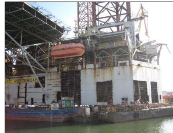
Replacement of Corroded Plates
