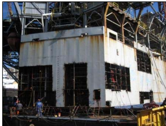
Replacement of Corroded Plates
