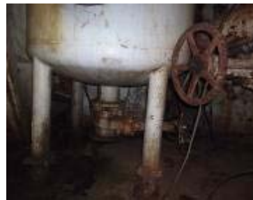
View on Supporting Legs of Existing Mud Gas Separator
