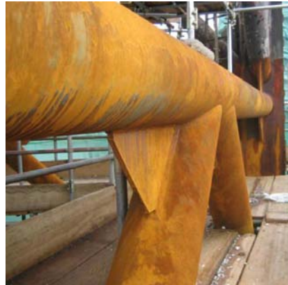
General View of Truss
